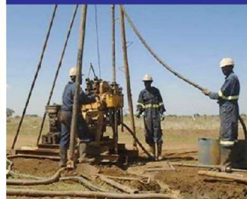
Soil Test and Foundation Analysis
